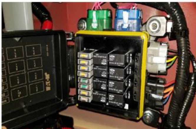
Figure 7.1.2.2: Overhead Switches dedicated electrical center.
